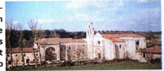
Exterior view of San Juan de Ortega
